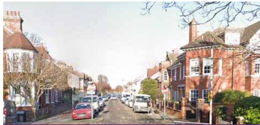
Shaftsbury Avenue, Bedford - very different approaches to the design of the way these opposite homes turn the corner but the overall scale is harmonious
