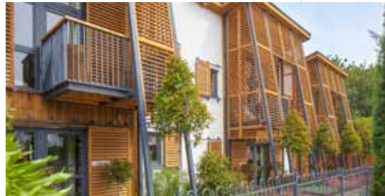
Climate change adaptation - external shutters to prevent overheating
