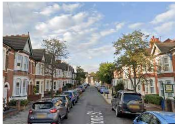
Gladstone Street, Bedford - homes that face onto each other create a strong sense of place and a well defined street
