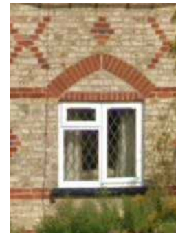
Yellow/red brick detailing on wall elevations
