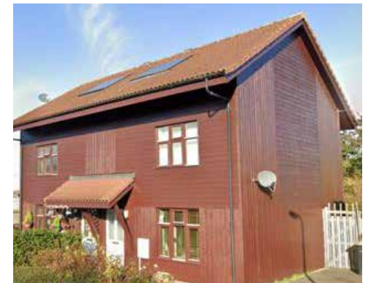
Maia Close, Bedford - entrance canopy mirrors main roof and is of appropriate scale and detail
