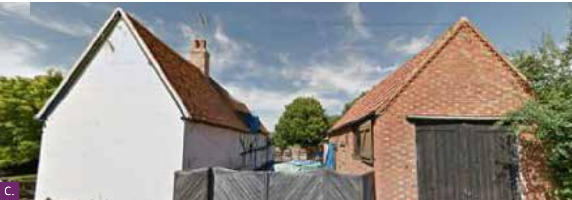
C. Chequerboard brickwork used to construct outbuildings, shops and terraced homes
