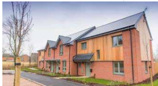
Sharnbrook, Passivhaus (13 dwellings) - consider Passivhaus and net zero standards for new homes
