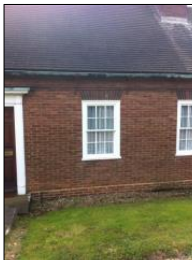
Fig. 65. 1956 phase of development, six over six sash window
