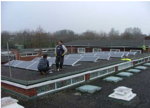
Solar PV panels being installed on Brickhill Lower School's roof
