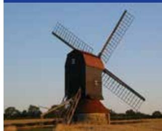
Constructed around a central post so that it can be turned to face into the wind, this impressive postmill was built in the 18th century and is the only complete windmill left in the county.
