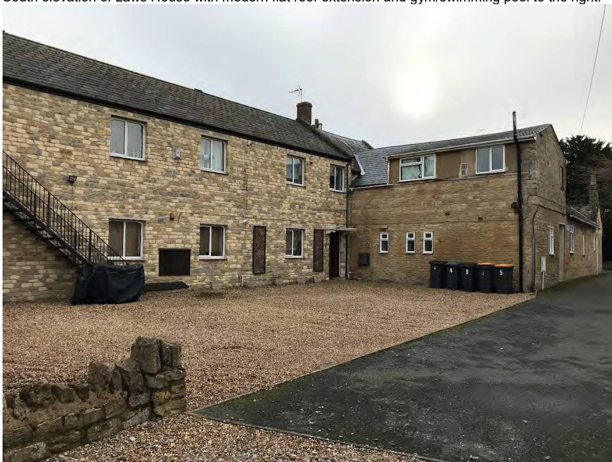
View from north west (end of Laws Close). On the left is the converted former hotel rooms (4 and 5 Laws Close), and on the right is the west elevation of Laws House and the access to Laws Close.
