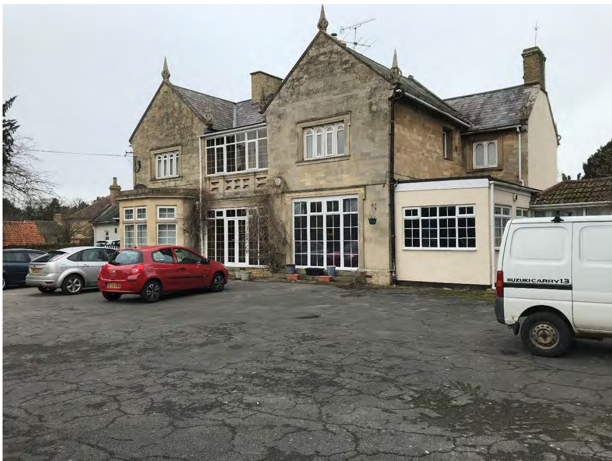
South elevation of Laws House with modern flat roof extension and gym/swimming pool to the right.
