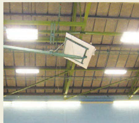
Biddenham Upper School lighting project replacing t12 with T5 lights.
