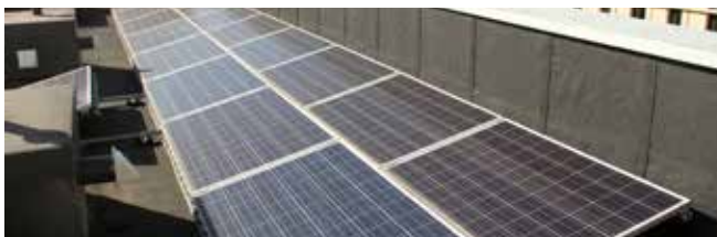
Extensive PV array hidden by parapet edge
