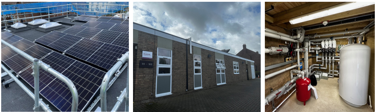
Photos: Brookside Care Home Energy Efficiency measures installed in 2024
