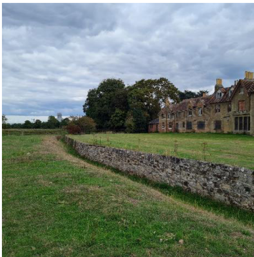
Figure 10 The grade II listed ha-ha wall to the north west of the New Manor House, designed to facilitate views towards the parkland and possibly the Church and 18th century manor beyond.
