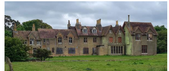
Figure 17 The west elevation of the New Manor House. The building's remodelling is attributed to the architect John Usher and is described by Pevsner as 'rambling'. The elevation is relatively plain in terms of detailing.
