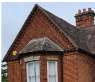
Figure 21 The 19th century addition to Lower Farmhouse, which utilises a similar dentil course within the gable end apex.
