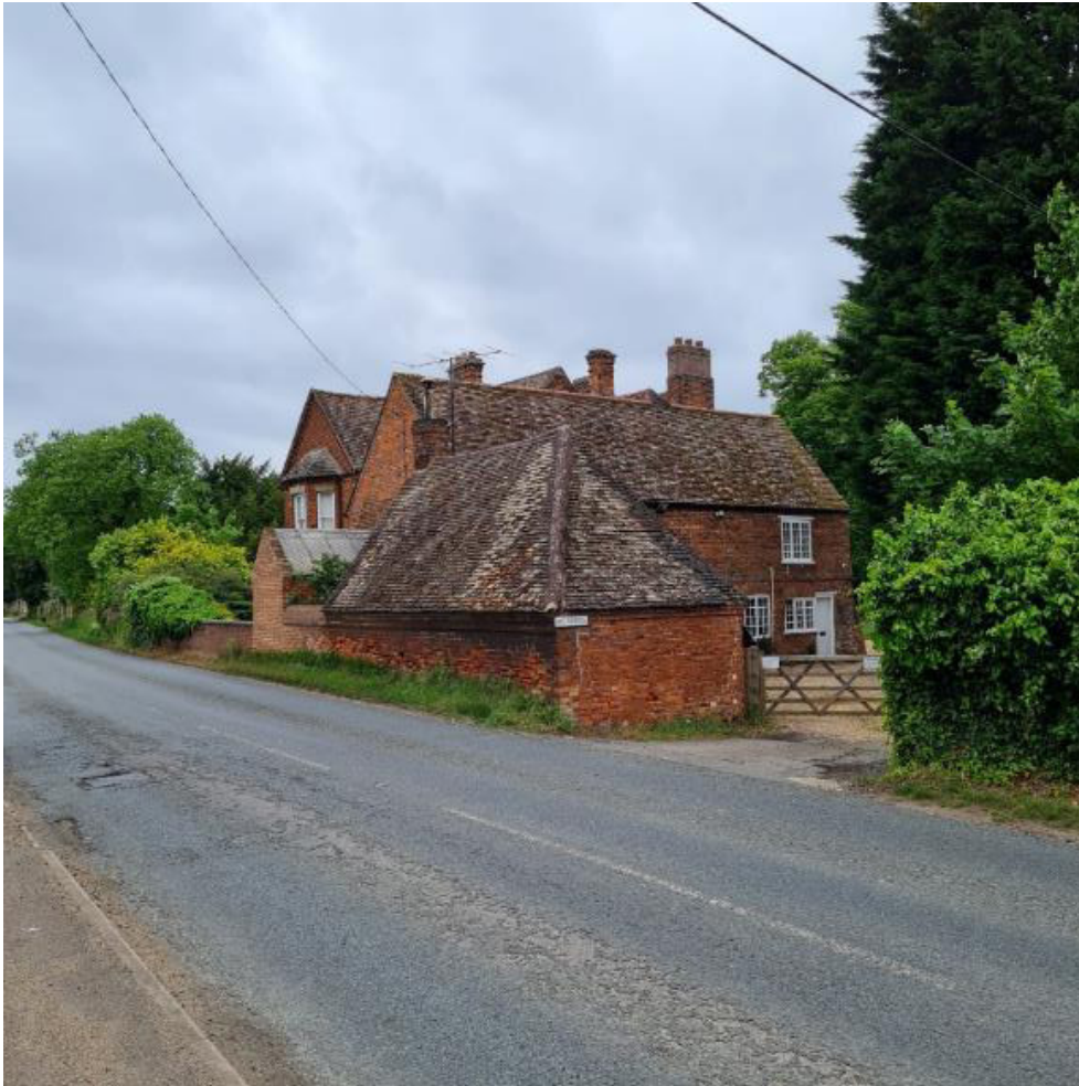
View 1 – View of Lower Farmhouse from Barford Road, taking in the varying roofscapes and phases of development.
