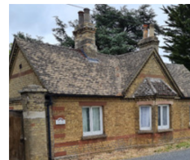
Figure 20 The principal elevation of South Lodge, with dressed stone detailing and a dentil course to the eaves and verges.
