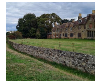
Figure 26 The ha-ha wall running to the west of New Manor House.
