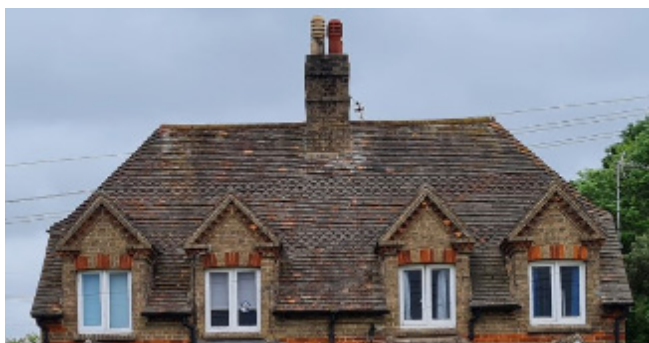
Figure 24 Fishscale tiles used at 7 and 8 The Cottages.
