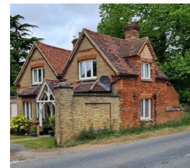
Figure 15 North Lodge is built from both red and buff brick. The red brick utilised for the east elevation harmonises with the red brick boundary wall which continues northward.
