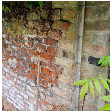
Figure 16 18th century red brick alongside modern buff brick in the former kitchen garden wall for the 18th century manor, now within the garden of the Dower House.
