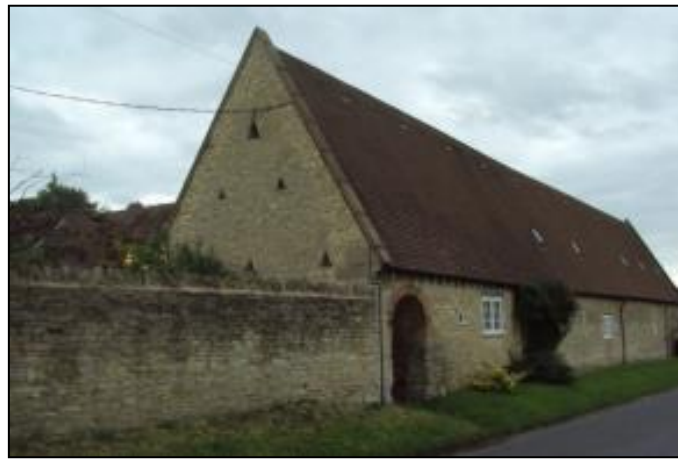
Fig. 16. West Farm Barn
