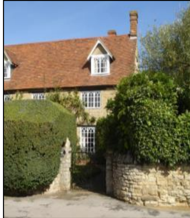
Fig. 31. Stone walls and gate piers at Grove Farmhouse, 18 Main Road
