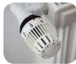
Install and correctly use a room thermostat and thermostatic radiator valves. Set them to the level you want for the room. A lower setting uses less energy.
