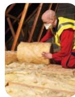
Up to 25% of the heat in your property could be escaping through the roof if it is not insulated. If your property has an accessible loft with no damp or condensation problems, then loft insulation should be easy to install either by DIY or by contacting an installer.
