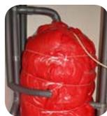
Insulate your hot water cylinder – a well fitted tank jacket could save around £20 - £30 a year, more if the water is heated electrically. Insulating the hot water pipes will save more energy, and can help the taps to run hot more quickly.
